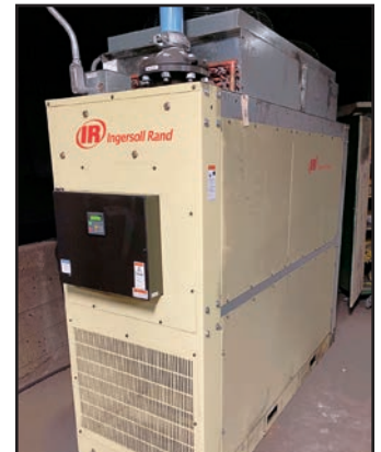
INGERSOLL RAND D4080INA400 REFRIGERATED AIR DRYER
