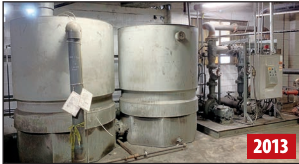
ADVANTAGE TTK-3000-3P WATER COOLING SYSTEM
