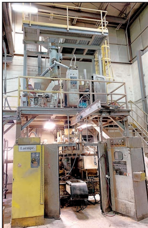
LAEMPE L-20 COLD BOX CORE CELL
