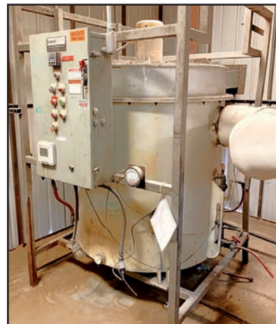
INTEREL MS-2500 SCRUBBER
